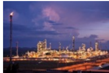
Dung Quat oil refinery
