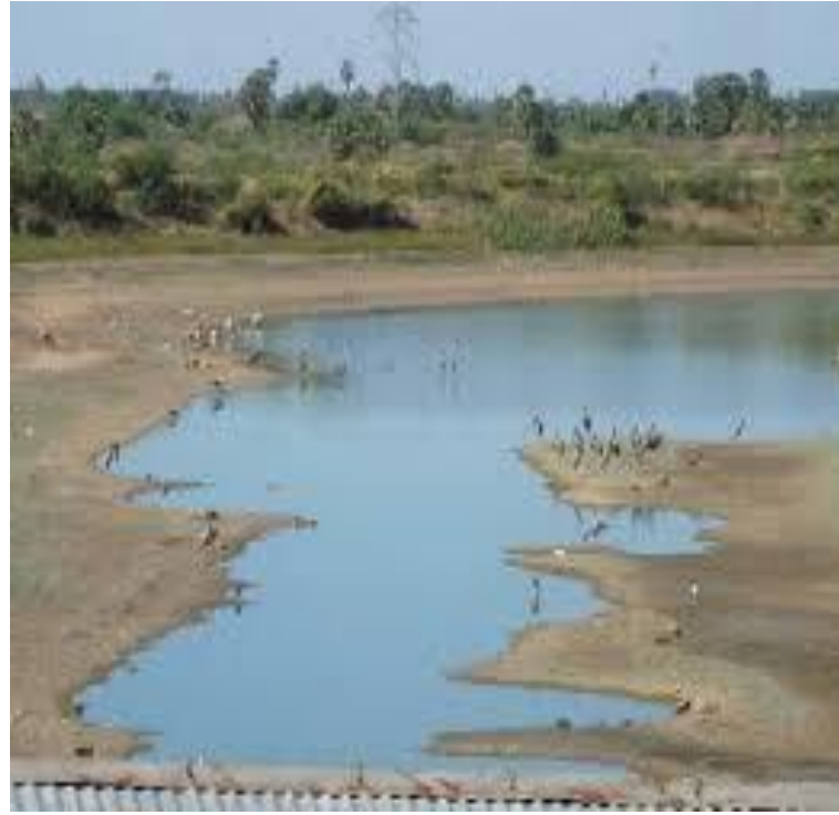
Siltation and Reduced Water Carrying Capacity
