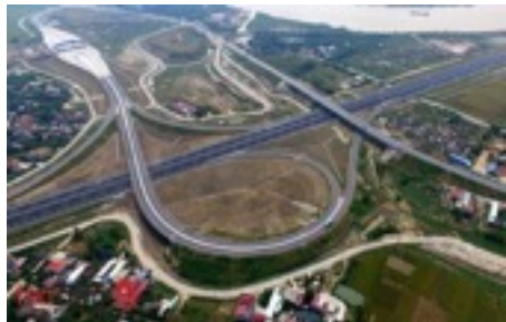
Ha Noi – Hai Phong expressway
